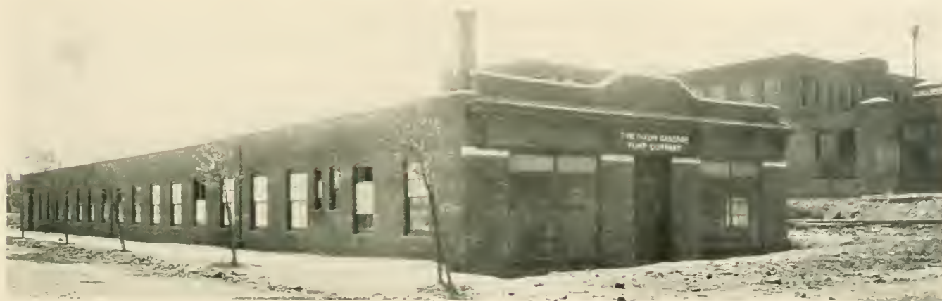
THE DIXON CASCADE PUMP CO., BADGER AVENUE AND RUNYON STREET.
